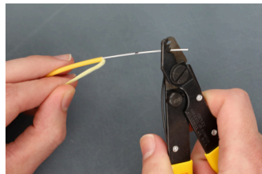
Step 6: Strip off the 900µm tight buffer coating all the way back to the marked spot. Do this in small sections at a time to avoid breaking the fiber. Ensure that the acrylate coating is completely off the fiber.
